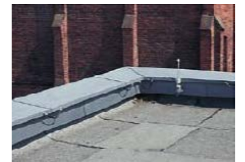
Wall Coping (with an inward slope ≥3°)
