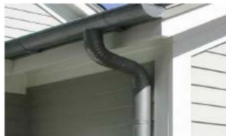
External Gutter with Downpipe
