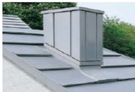
Chimney Flashing
